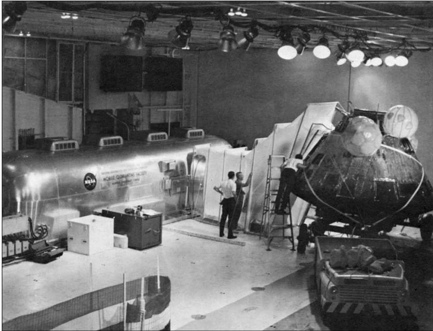
Figure 7-8.- Installation of the tunnel between command module and quarantine facility.
