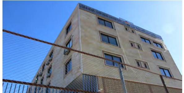
Burj El-Chamali Municipality © Photo: Maya Majzoub, UN-Habitat, 2016.
