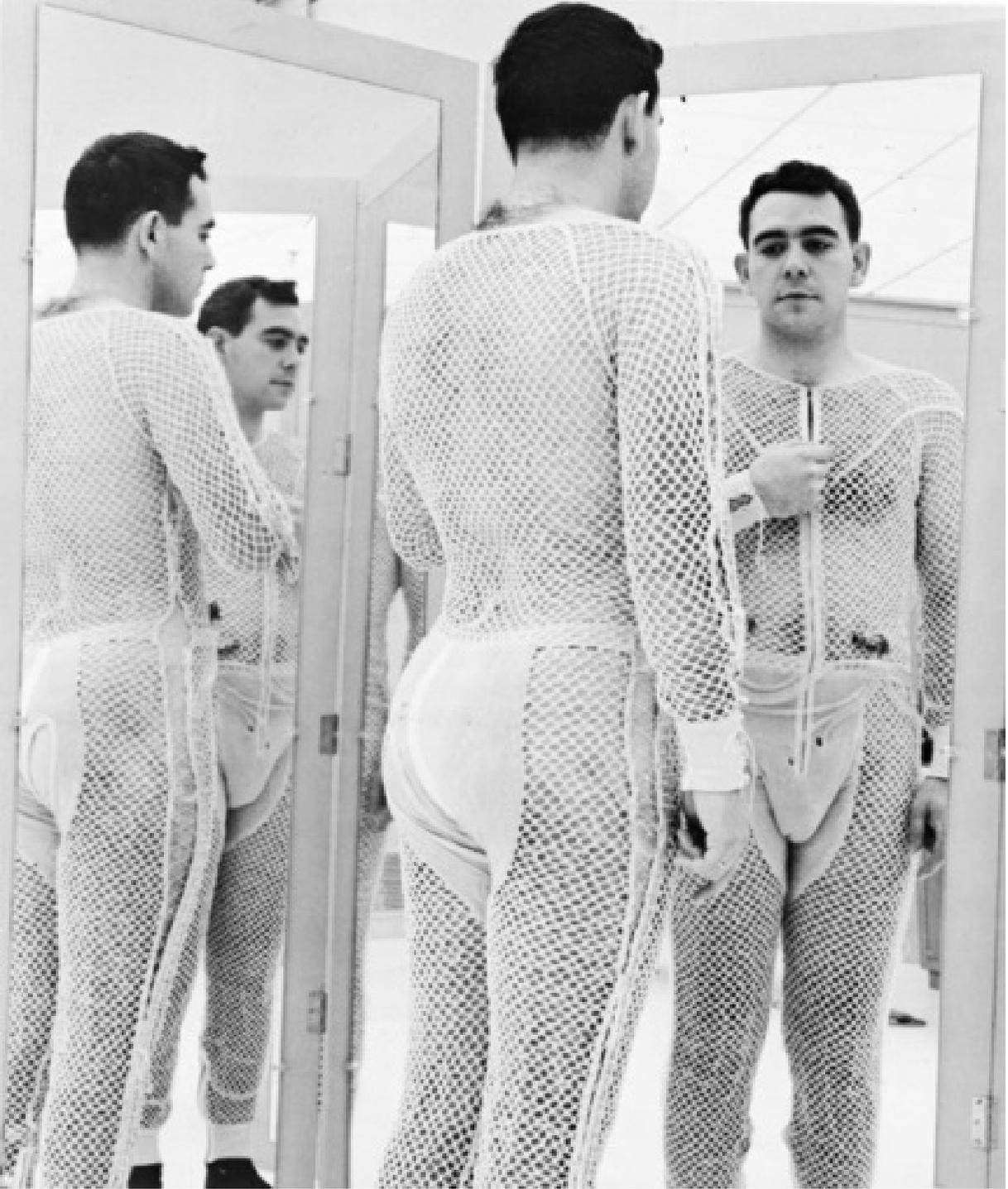
Figure 12 HSD Engineer Mark Britanisky Demonstrating The CG2 Liquid Cooling Garment (Courtesy United Technologies Aerospace Systems)
