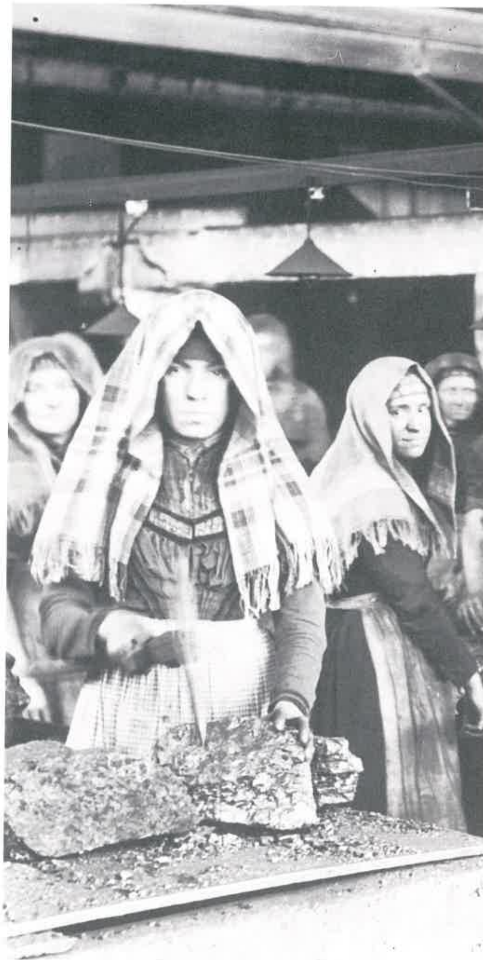
56 The screens at Chanters Pit, Atherton, Lancashire, 1905. The mesh screens separated small from large coal. The woman on the left is using a pick to break off dirt
