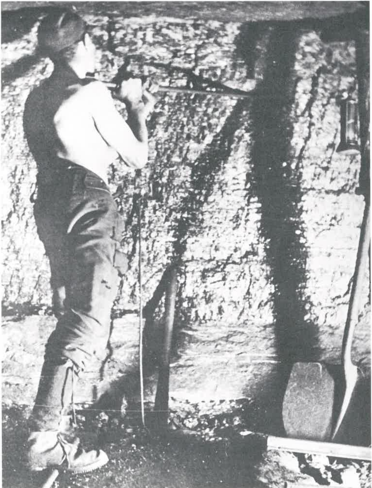
2 A miner using the most primitive form of hand-drilling at Douglas Bank Colliery, Wigan. The drill was simply a steel rod with a sharpened end. After every three inches or so, the scraper, next to the pick, was inserted to pull out the dust
