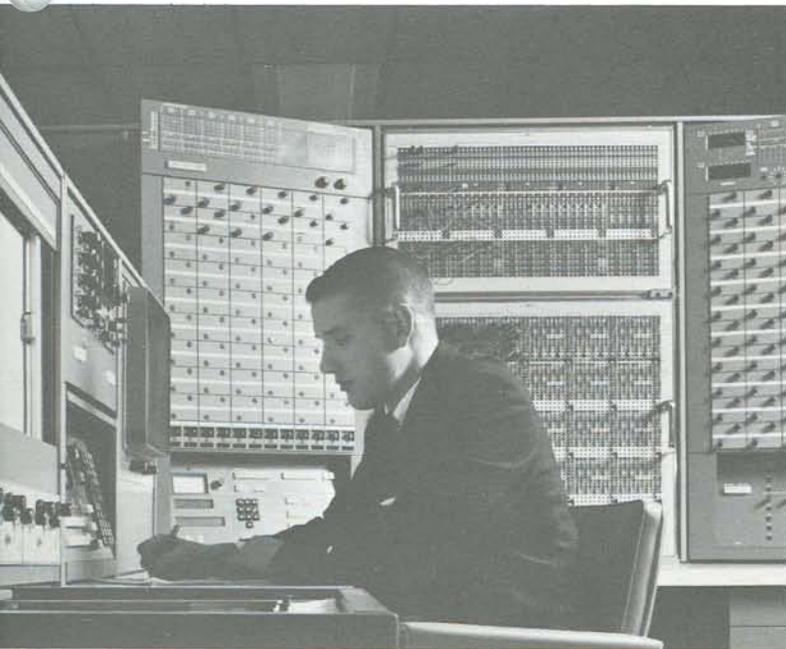
The Console of the EAI 8800 System is a self-contained computing center with programming, control, and computing components all housed within its three-bay structure. It combines ease and flexibility of programming with multi-level analog and logic control of its large-scale computing capacity. Detailed consideration has been given to human-engineering as an operator-oriented system, with emphasis placed on convenience and efficiency of operation.
